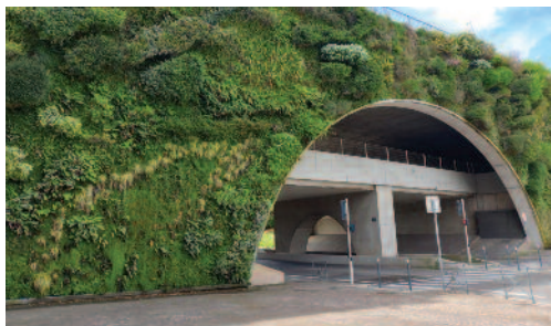
Living bridge, Aix-en-Provence
